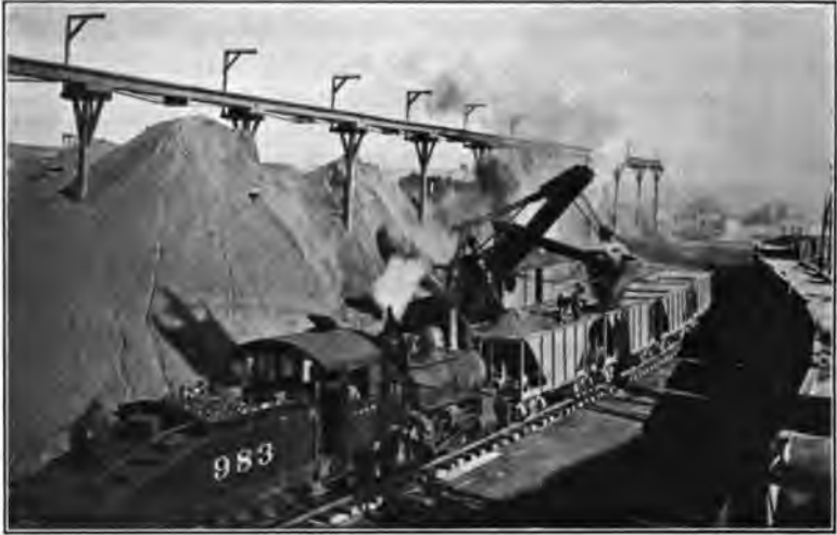
ONE-LEG TRESTLE, COLBY MINE. LOADING STOCKPILE
